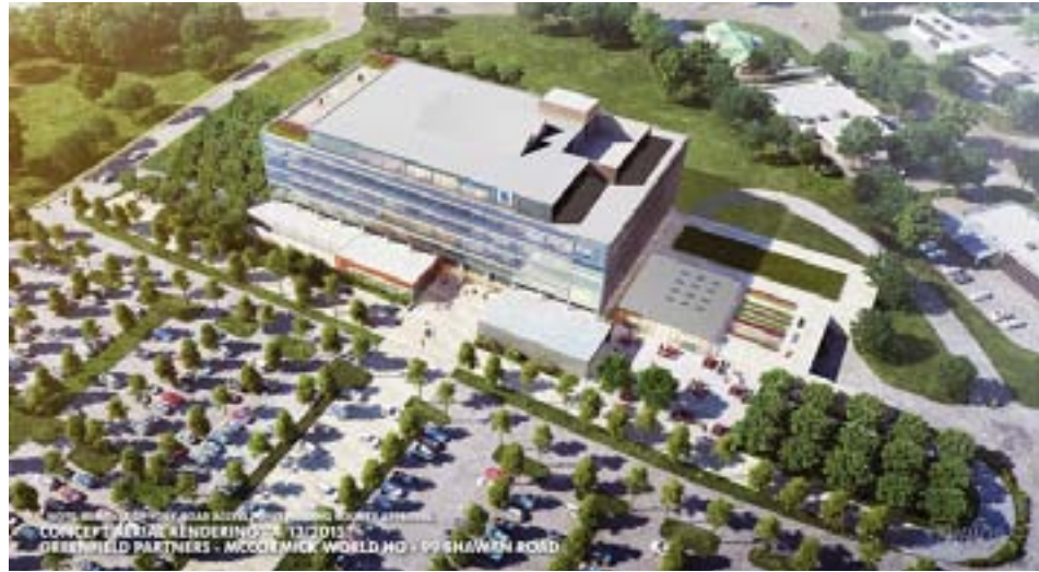
The new McCormick campus sits at the southwest corner of Shawan/York roads on 20 acres of land. Enhancements include a 339,000 square-foot six-story building. Photo: McCormick & Company
