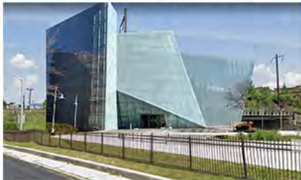
WEST BALTIMORE MARC STATION (front perspective) - building-only cost estimate: $17 million - $94 million currently budgeted for station and track - presumed funding with B&P tunnel replacement
