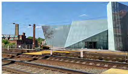
WEST BALTIMORE MARC STATION (track perspective) - conceptual rendering of new marquis, multi-modal station replacement station planned for track realignment - would be ~ 60,000 sq. ft. with track access on second level
