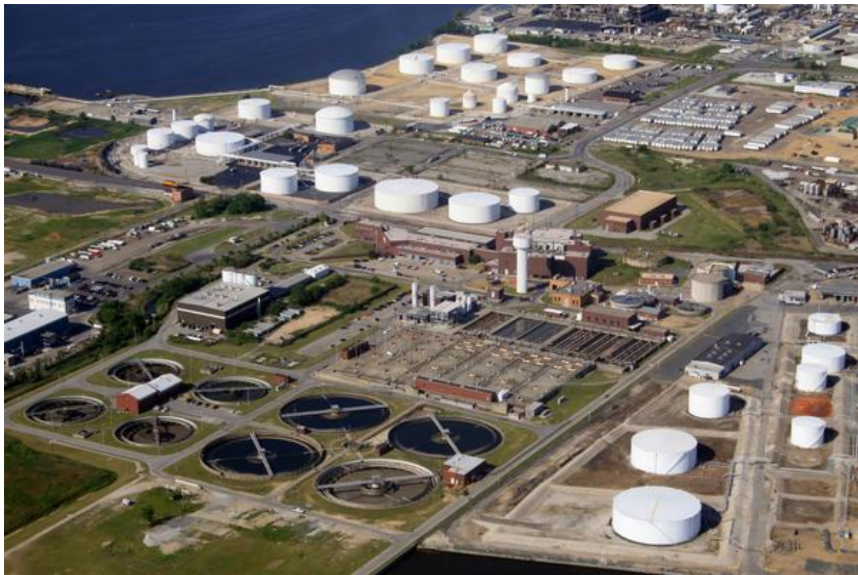
Figure 22. Back River Wastewater Treatment Plant.
