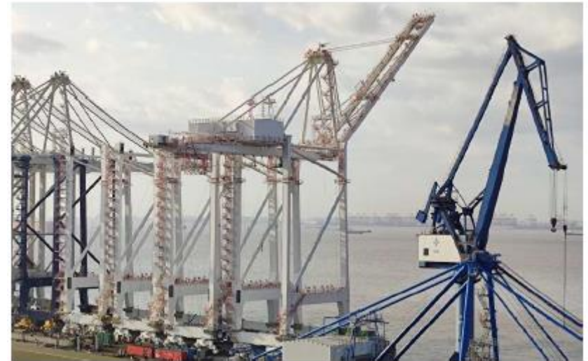
Description: Portal beam #1 is in 4-side fit-up process
