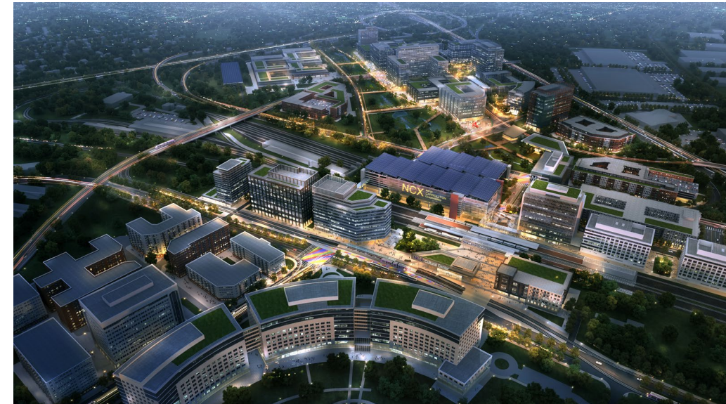
WMATA New Carrollton Expanded Joint Development spurred by New Garage and Bus Facility
