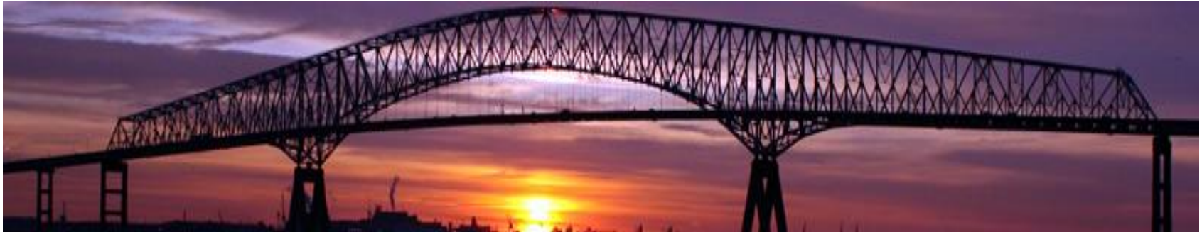
March 23, 1977: 1.7 mile-long Key Bridge opened over the Patapsco River as part of I-695
