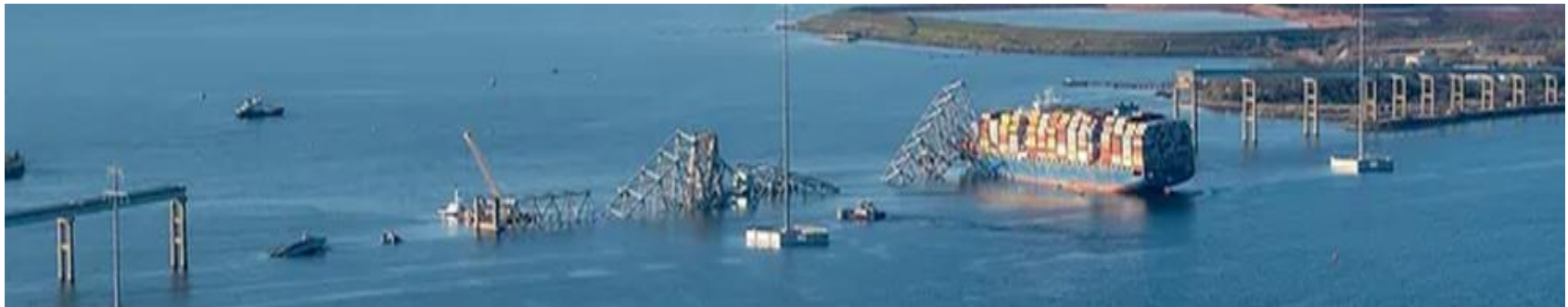
March 26, 2024: Cargo ship leaving the Port of Baltimore strikes the Key Bridge causing its collapse
