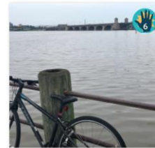
Hanover street bridge - built in 1916 - looking good (Baltimore, MD) S Bailey
