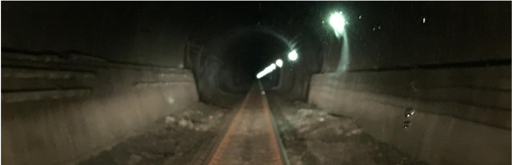
Inside Howard Street Tunnel
