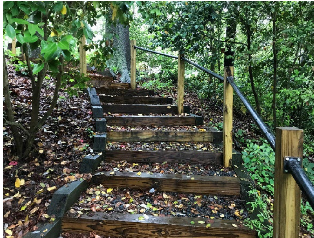
Anne Arundel County - Woodland Gardens Trail Restoration, London Town Foundation
