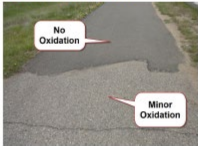
Figure Two: Oxidation
