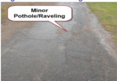
Figure Three: Raveling
