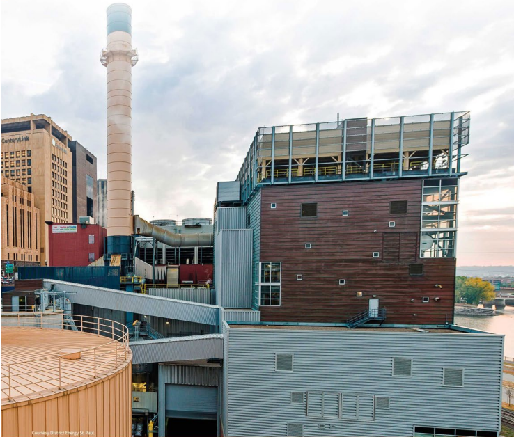
At the District Energy St. Paul location along the Mississippi River in downtown St. Paul, a significant amount of activity takes place on a very small parcel. This central facility integrates biomass-fired combined heat and power, thermal storage, and the primary heating and cooling production for this system.
