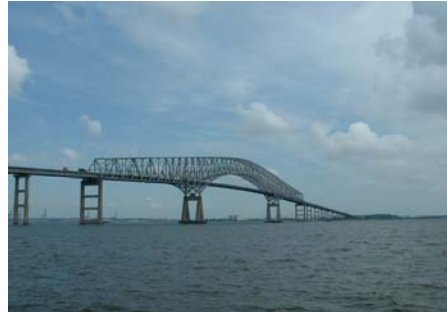
Francis Scott Key Bridge
