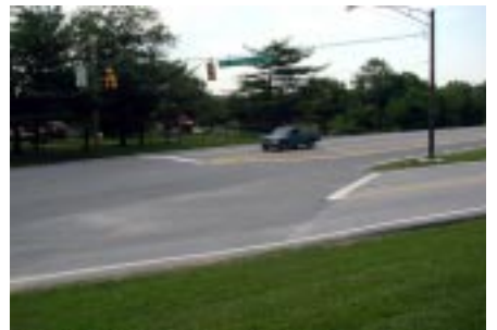
(Above) Sidewalks are missing on all approaches to the school. Traffic speeds are high, and turning movements are complex. Children cannot see the signals, and pedestrian signals are missing. This intersection may model well for a roundabout. Sidewalks are needed to area housing and other destinations.
